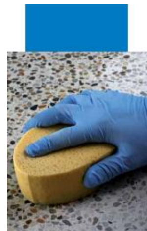
Dampening the surface with a sponge
