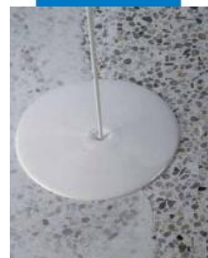
Application of Ultratop Stucco
